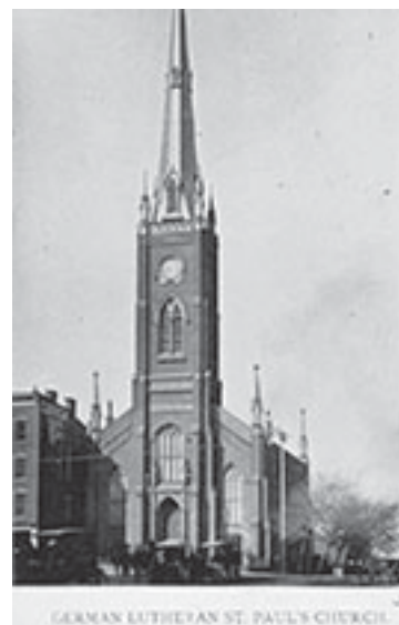
St. Paul's Ev. Church
